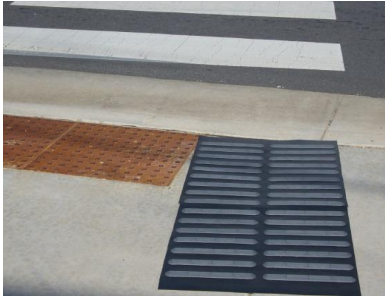
Figure 3. Photo of a guidance surface with raised bars perpendicular to the direction of travel across the crosswalk (Bentzen et al. 2017).
